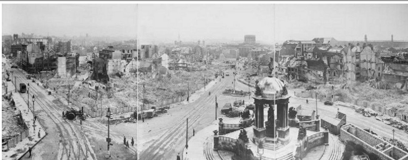
Bomb Damage after the May Blitz. The Custom House on the skyline had to be demolished.
